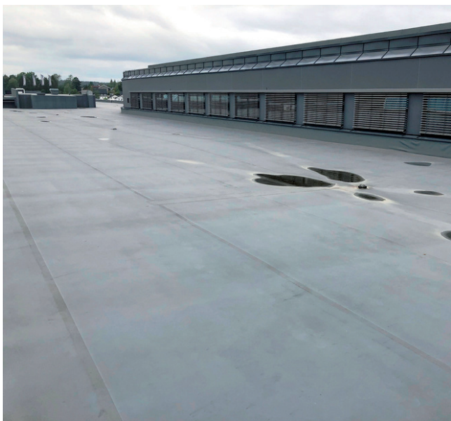
Figure 6: On the roof, there isn't much to see.
