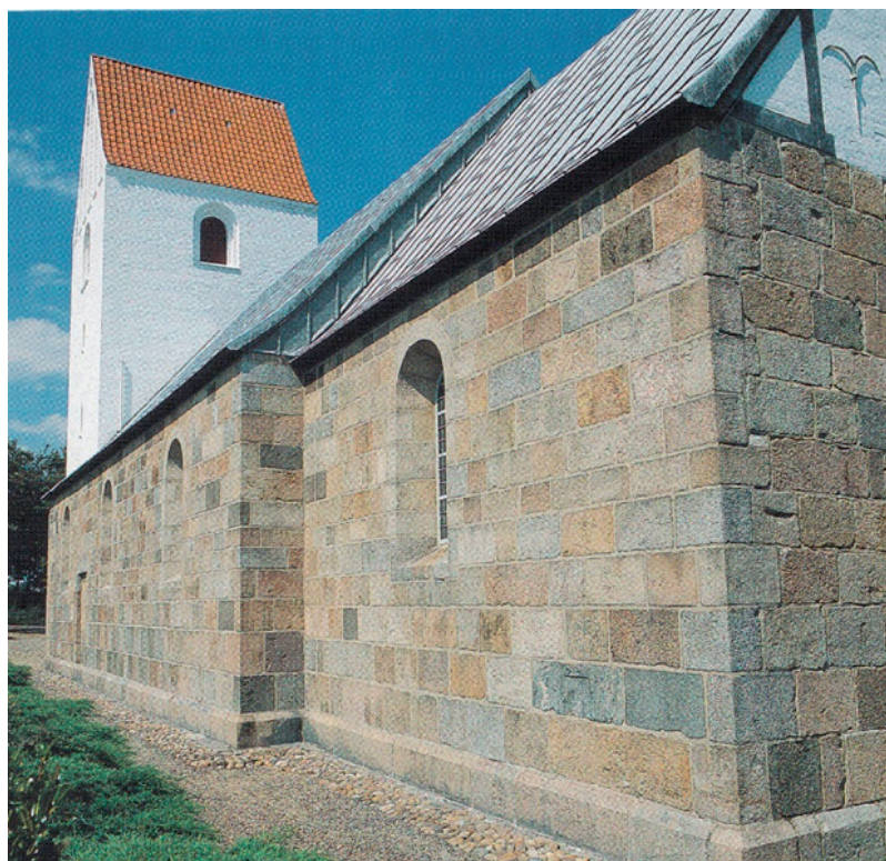
Figure 3: “Asp Kirke”, Jutland, typical medieval Romanesque church illustrating the diverse assembly of hewn rock types. Note later improvement (enlargement) of windows, later lead roofing and addition of a bell tower.
